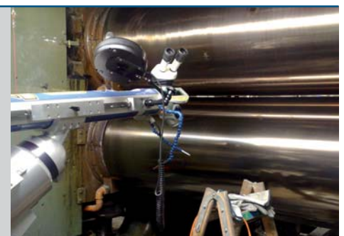
Repair welding on roller (Photo: tcms, Gummersbach)
